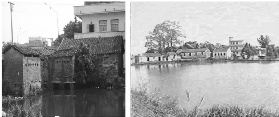
Appendix 2. Toilet reconstruction with sanitary toilets
